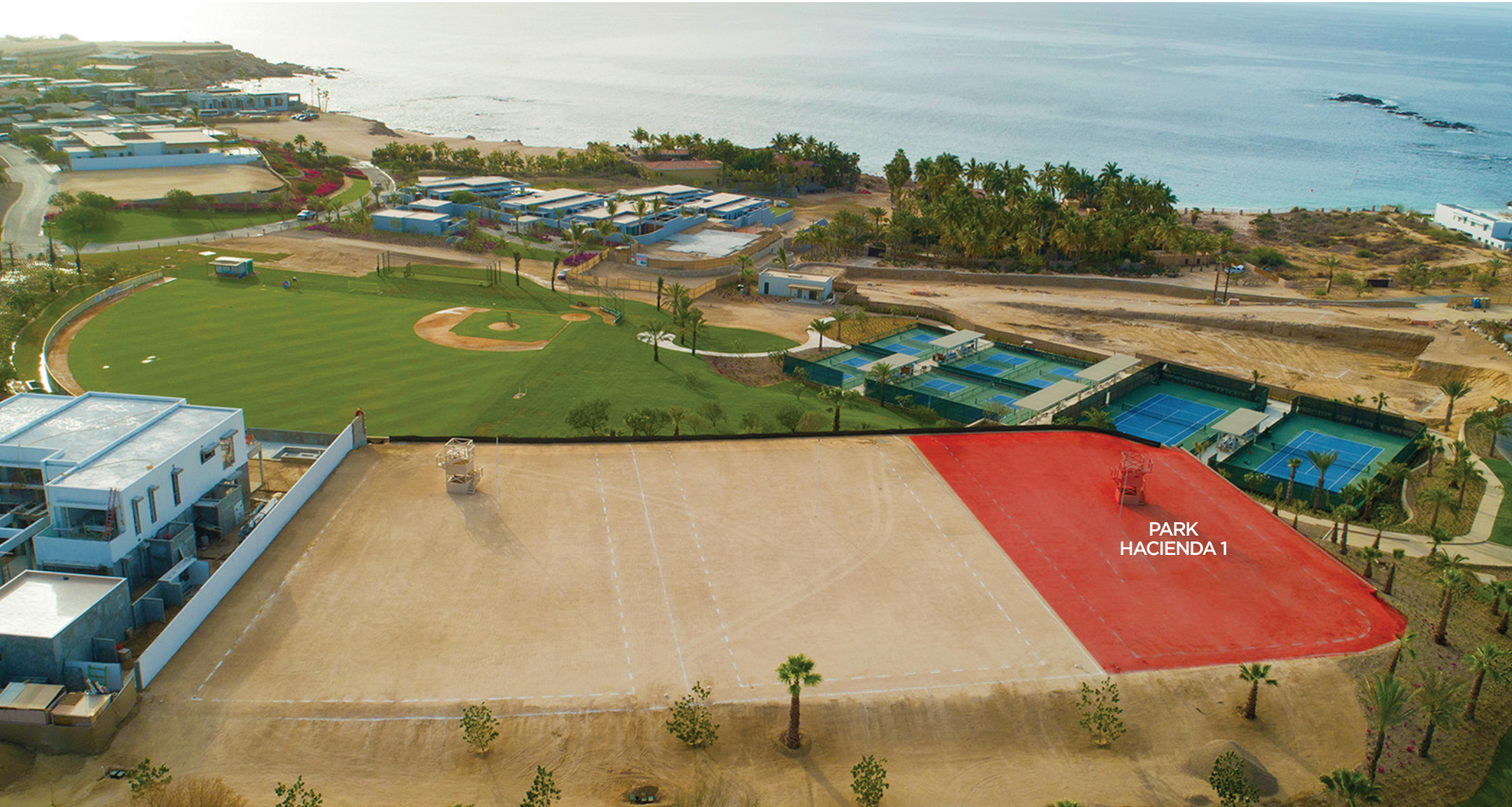
Aerial View of Park Hacienda Neighborhood
