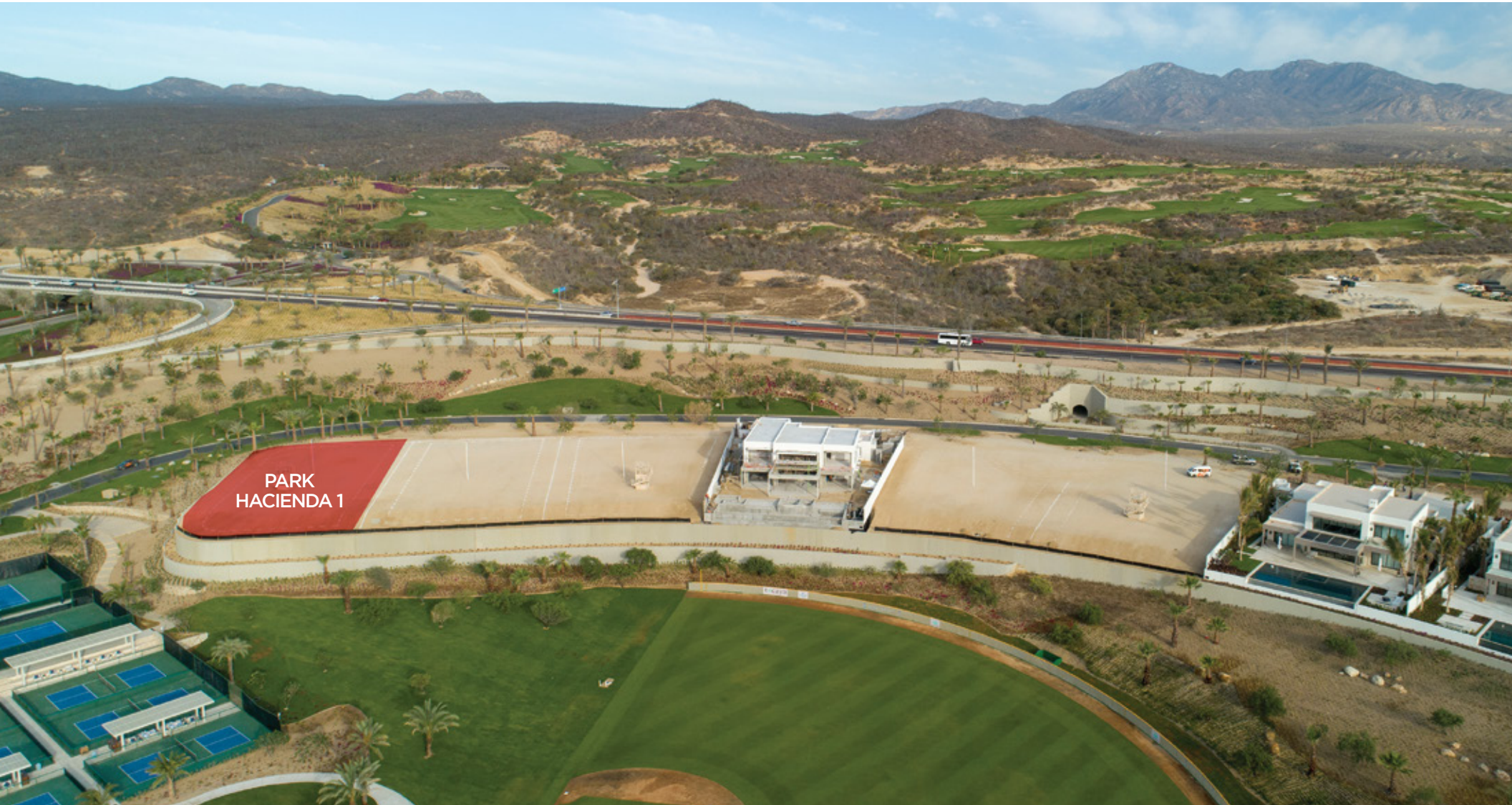
Aerial View of Park Hacienda Neighborhood
